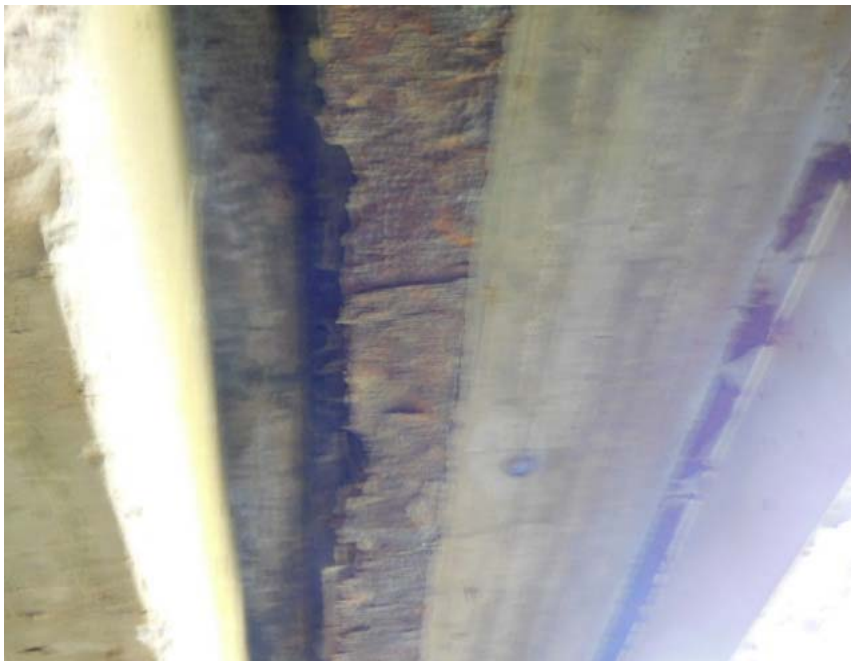
SPAN # 1 STEEL I BEAM "H" HEAVY CORROSION
