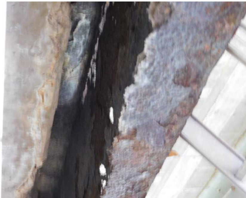
SPAN # 1 HOLE IN STEEL I BEAM "H"
