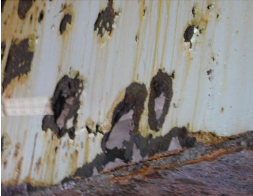
SPAN # 1 HOLE IN STEEL I BEAM "H" & HEAVY CORROSION
