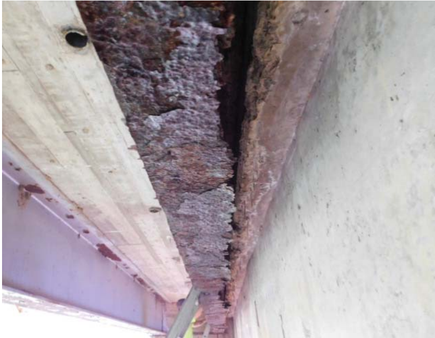
SPAN # 1 STEEL I BEAM "H" HEAVY CORROSION
