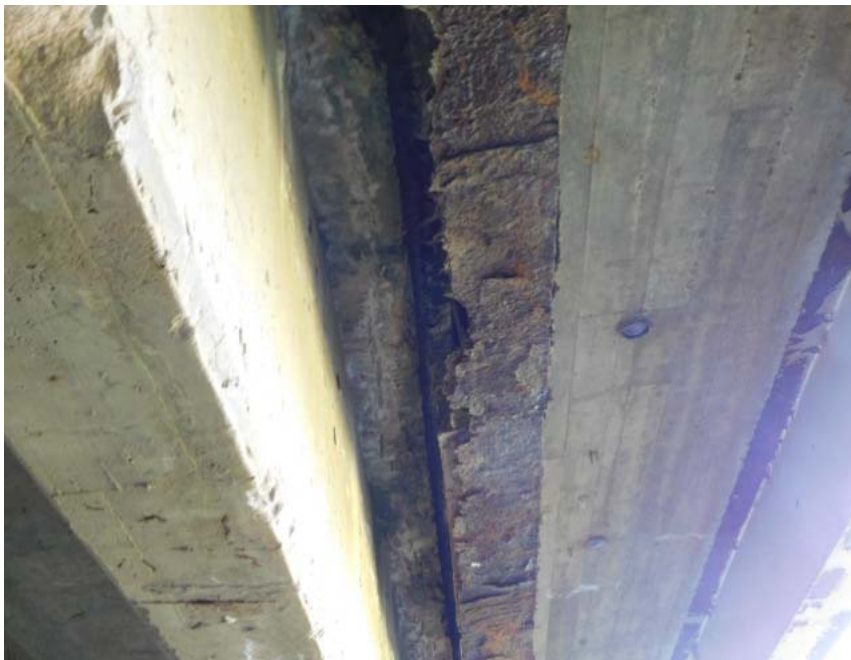
SPAN # 1 BOTTOM DECK SPALLING
