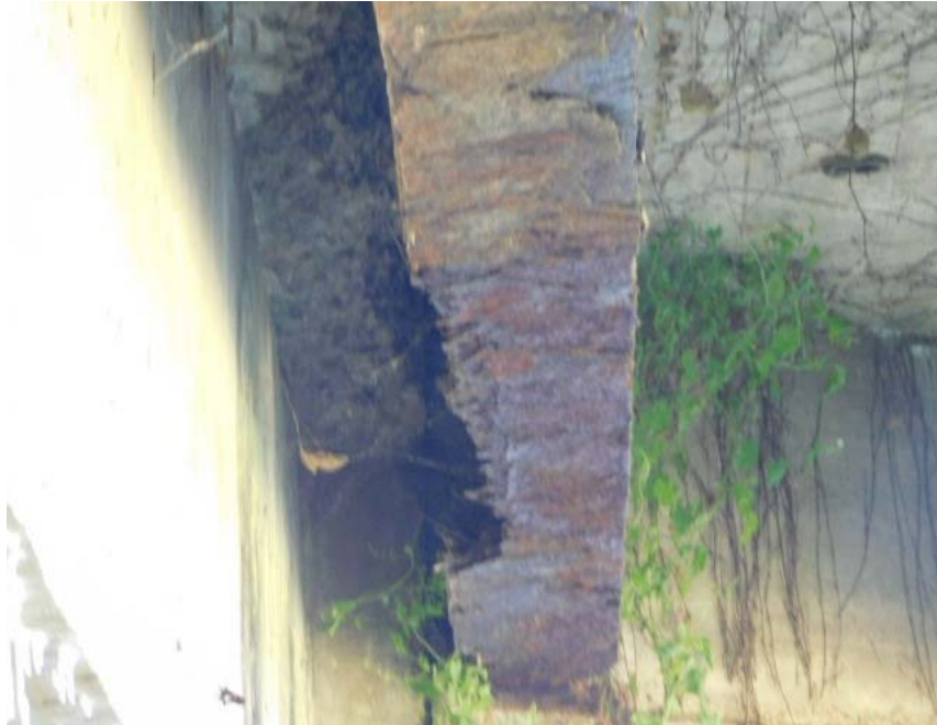
STEEL I BEAM "H" HEAVY CORROSION & SECTION LOSS
