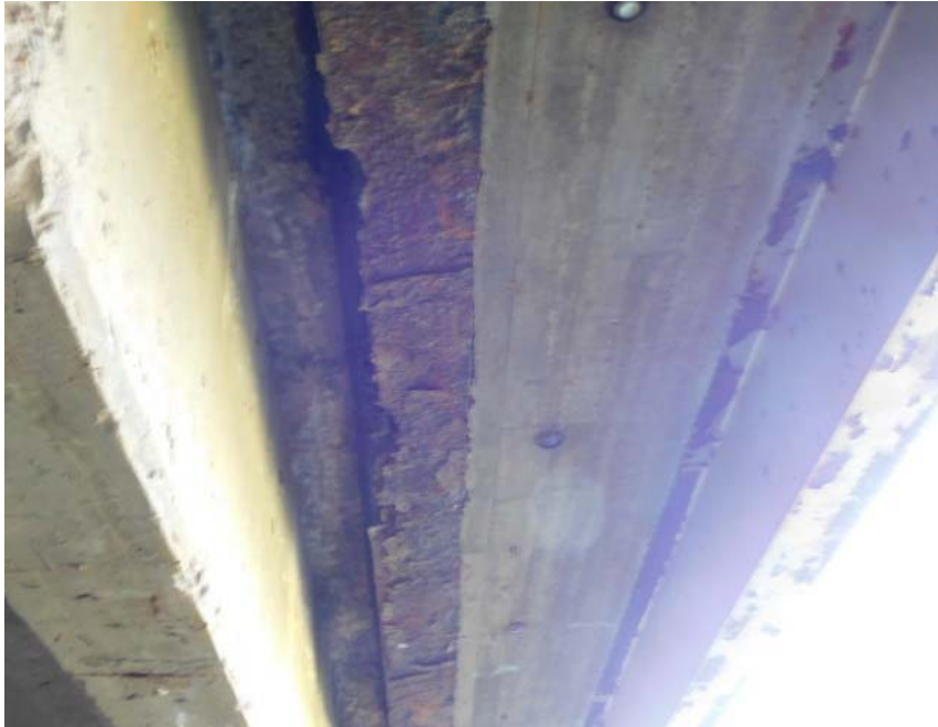
STEEL I BEAM "B" HEAVY CORROSION & SECTION LOSS
