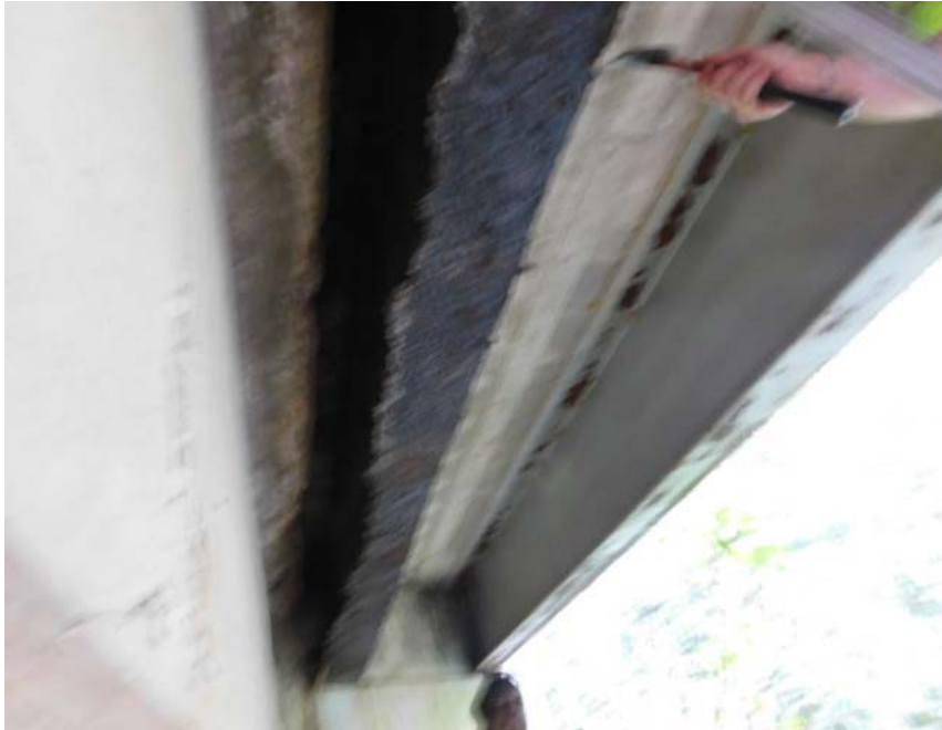
SPAN # 1 STEEL I BEAM "H" HEAVY CORROSION & SECTION LOSS
