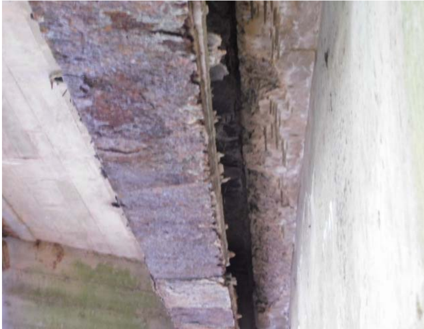
SPAN # 1 BOTTOM DECK SPALLING
