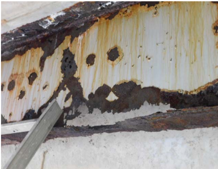
SPAN # 1 HOLE IN STEEL I BEAM "H" & HEAVY CORROSION
